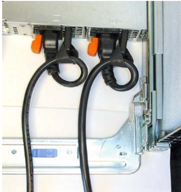
Figure 10. Proper PSU Cabling
